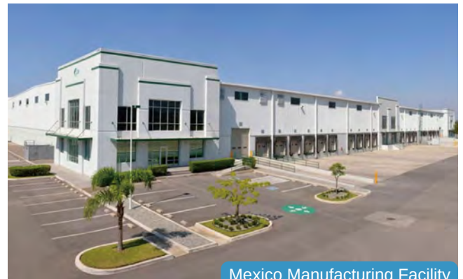
Mexico Manufacturing Facility
